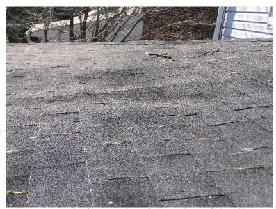
There are several low spots on the front porch roof where the roof sheathing has deteriorated. Water may collect in the low spots and eventually leak through the roof covering.
