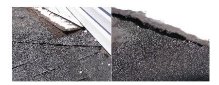
**Attention Needed** - Some portion of the roof flashing needs to have some repair. The flashing along the flat roof at the rear of the house is raised where it Page 30
