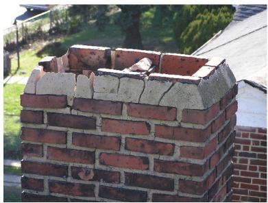
Action Necessary - The exterior stack has a condition that calls for repair. The top of the chimney is deteriorated and needs repair.
